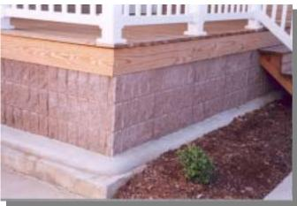
Concrete Footer: **Stone***Skirt* utilizes I-Beam technology which does not require the expense of a concrete footer.
